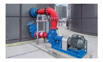
A liquid stream is drawn from the tank and pumped through a Hidrostal screw centrifugal pump to the mixing nozzle. In the nozzle, pressure energy is converted into kinetic energy, creating a lower pressure at the outlet that pulls in surrounding liquid. In the following mixing section, a flow profile forms that prevents particles from settling. This results in effective mixing of the medium through intense momentum exchange.
